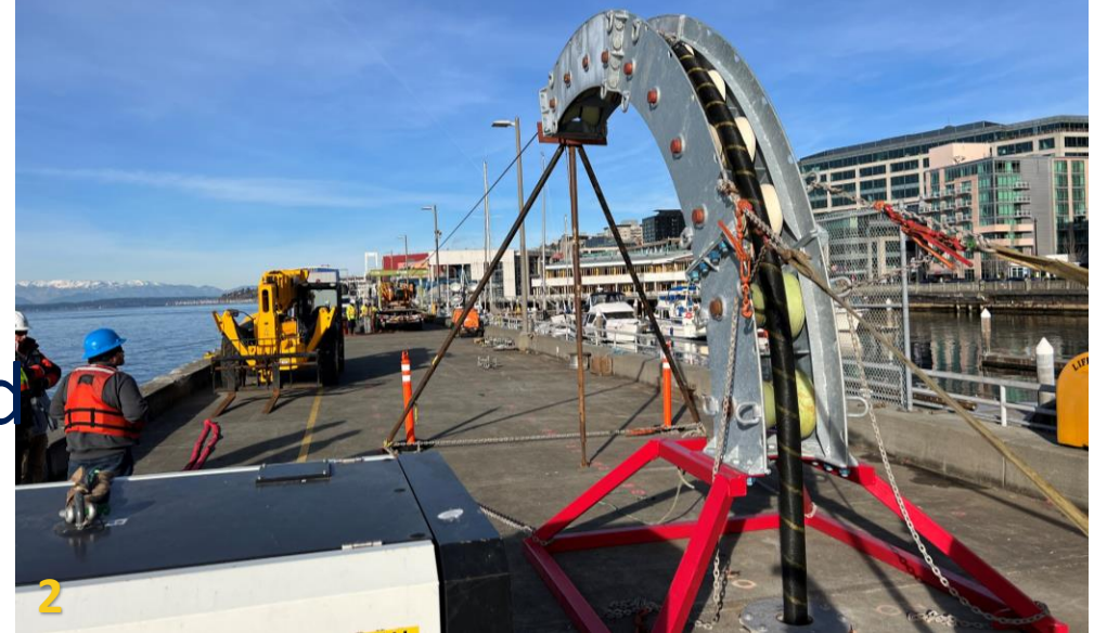
1. Jan 8, 2024: Submarine Cable Reel load onto barge at Terminal 46.
