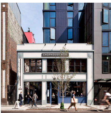
New development incorporates a historic facade and mid-block passageway. The two-story facade provides a transition from the taller building to a pedestrian scale and breaks up the building massing.
