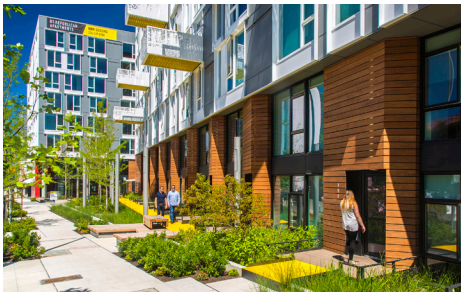
Frequent individual unit entries in the landscaped setback zone, and upper-level balconies provide an engaging edge.
