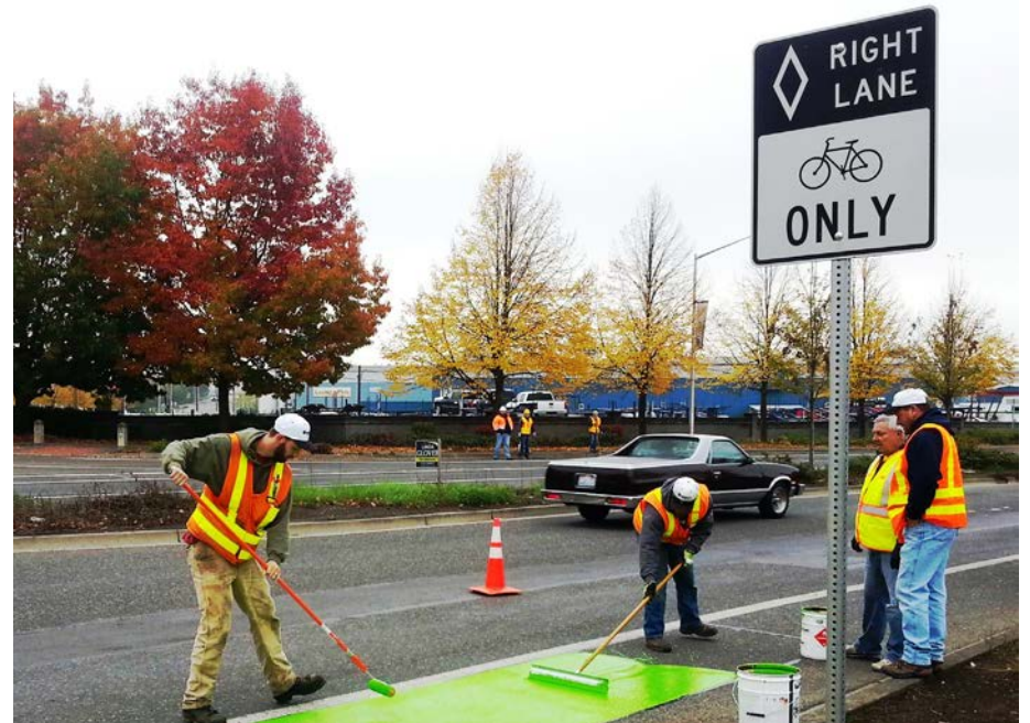
Crews painting a green bicycle lane
