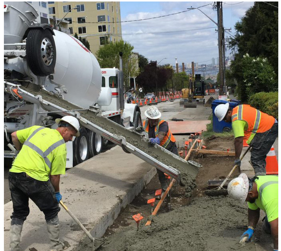
Construction crew at work in West Seattle
