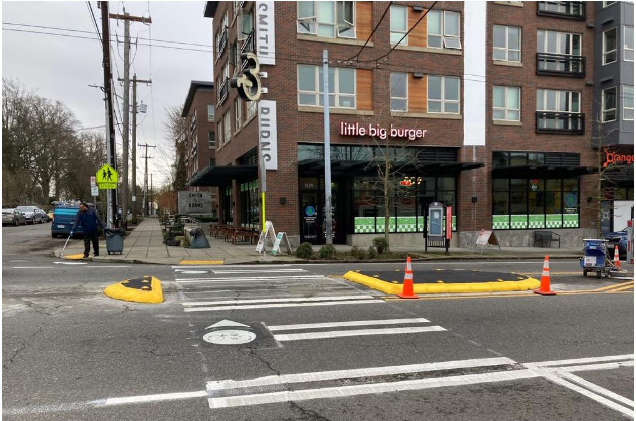
Program 25 – Crossing improvement at Interlake Ave N and N 45th St.
