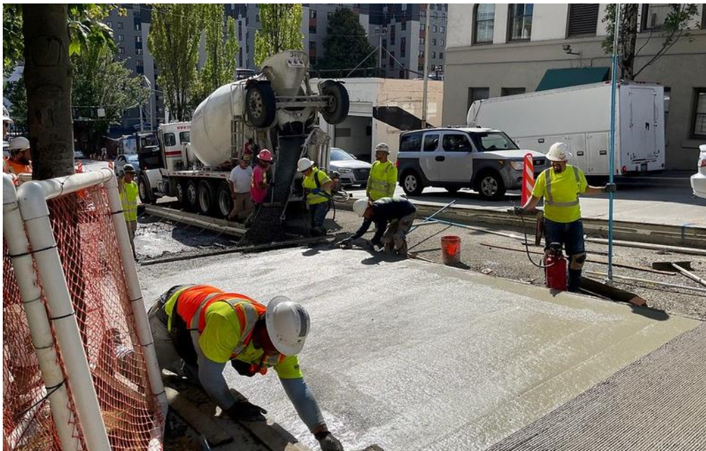
Repaving on E Madison St.
