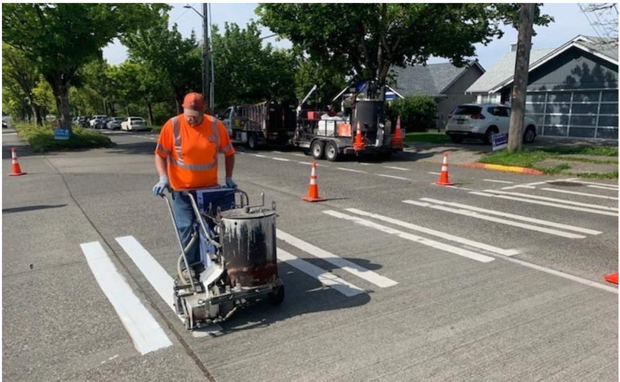
Program 3 - Remarking a crosswalk at 16th Ave SW and SW Findlay St.
