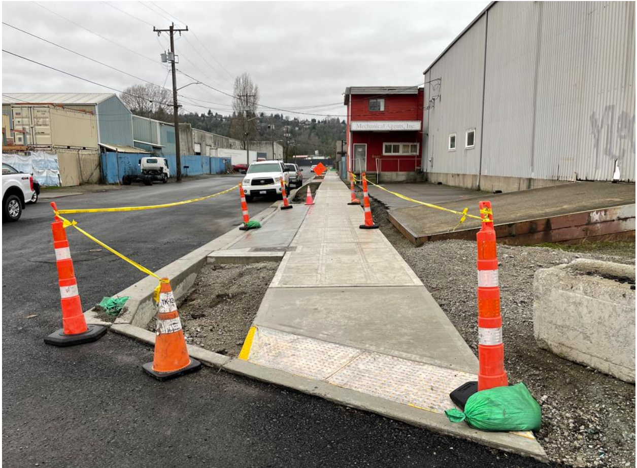
Program 17 – New sidewalks under construction in South Park.
