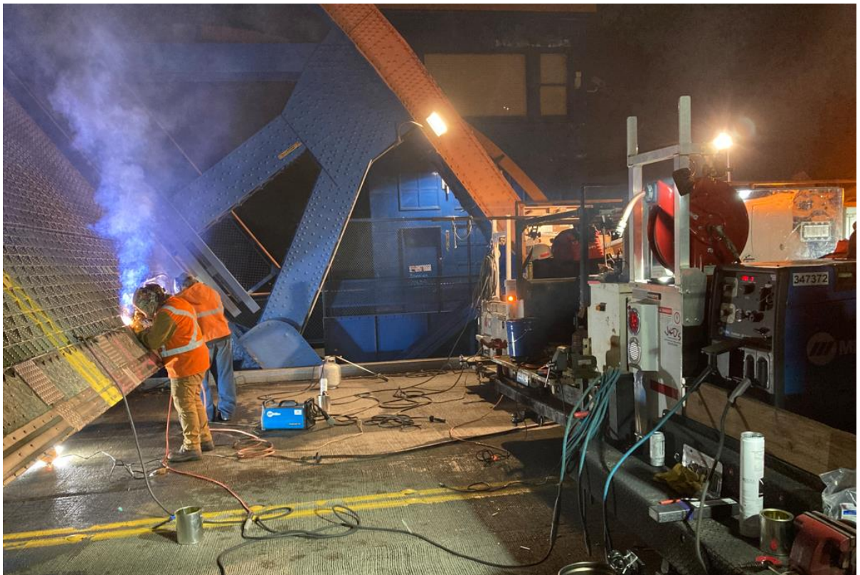
Program 11 - Deck welding repairs on the Fremont Bridge.
