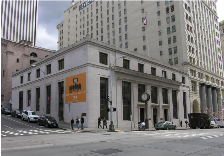
Seattle National Bank Building, 720 Second Avenue, 2012
