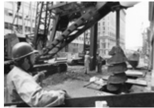
▲ Removing dirt from a hole for a soldier pile on Third Avenue near Yesler Way. April 30, 1987 Credit: MOHAI, Seattle Post-Intelligencer Collection
