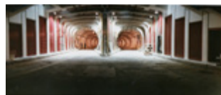
▲ Third Avenue tunnel entrance at University Street Station. April 1990 Credit: King County Office of Information Resource Management Printing and Graphic Arts photographs. Series 1147, Box 1, Folder 25.
