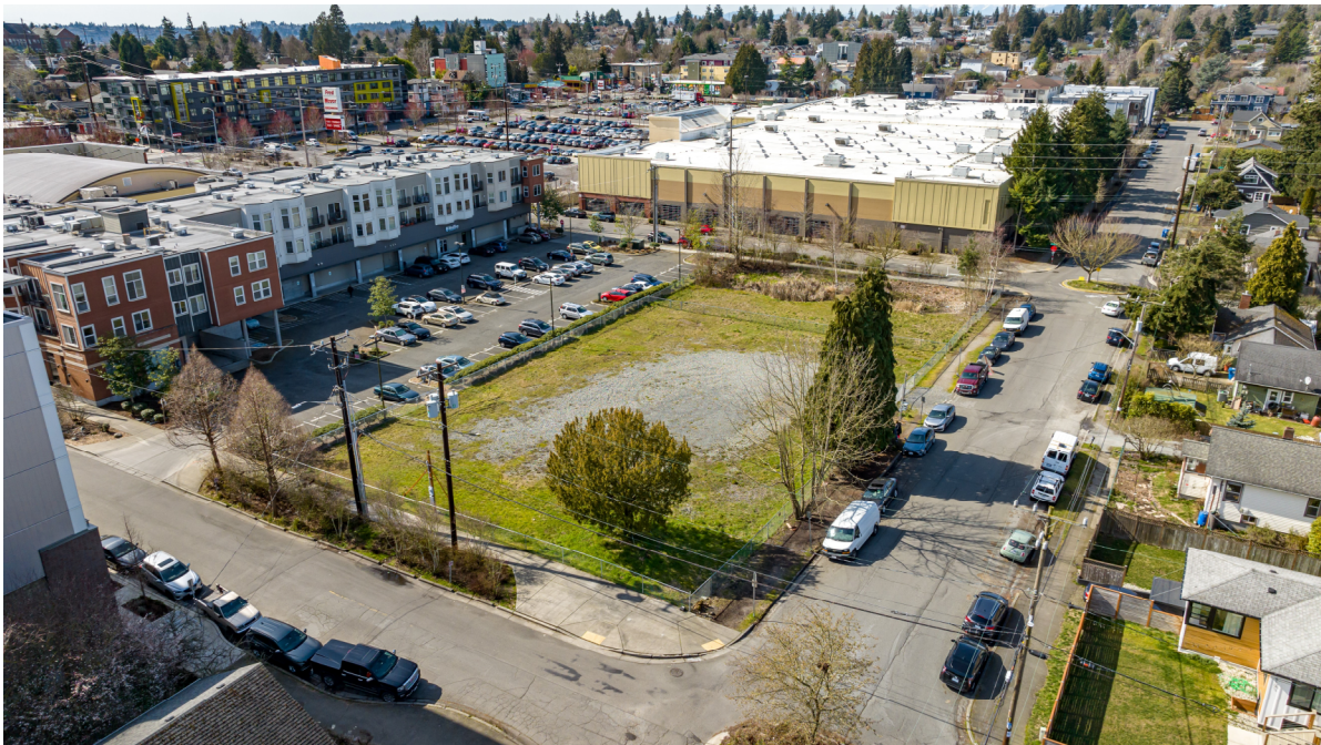
View of the Project Site from NE corner
