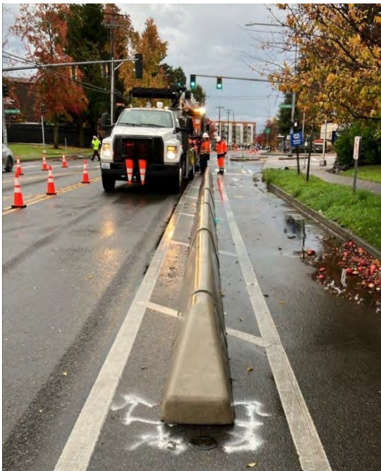
Toronto-style barrier being installed in Seattle
