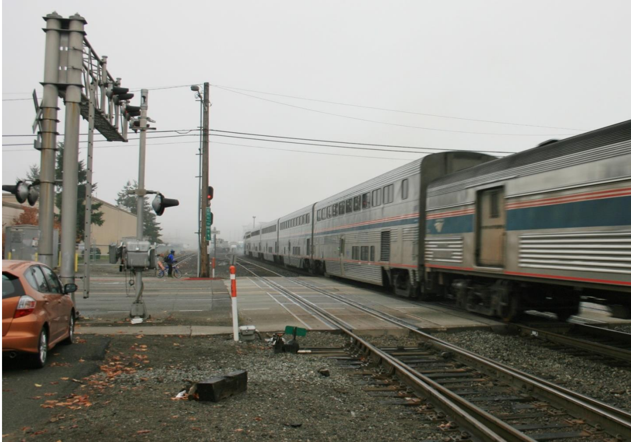
Figure 7: Current BNSF Rail Crossing at S Lander St
