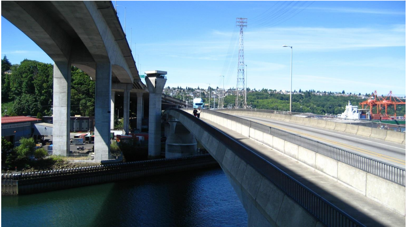
Figure 8: Lower Spokane St Swing Bridge
