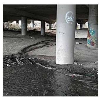
Seattle Fire Department response, shut down portions of the freeway, and resulted in visible but superficial damage to the concrete under-side of the interstate structure.
