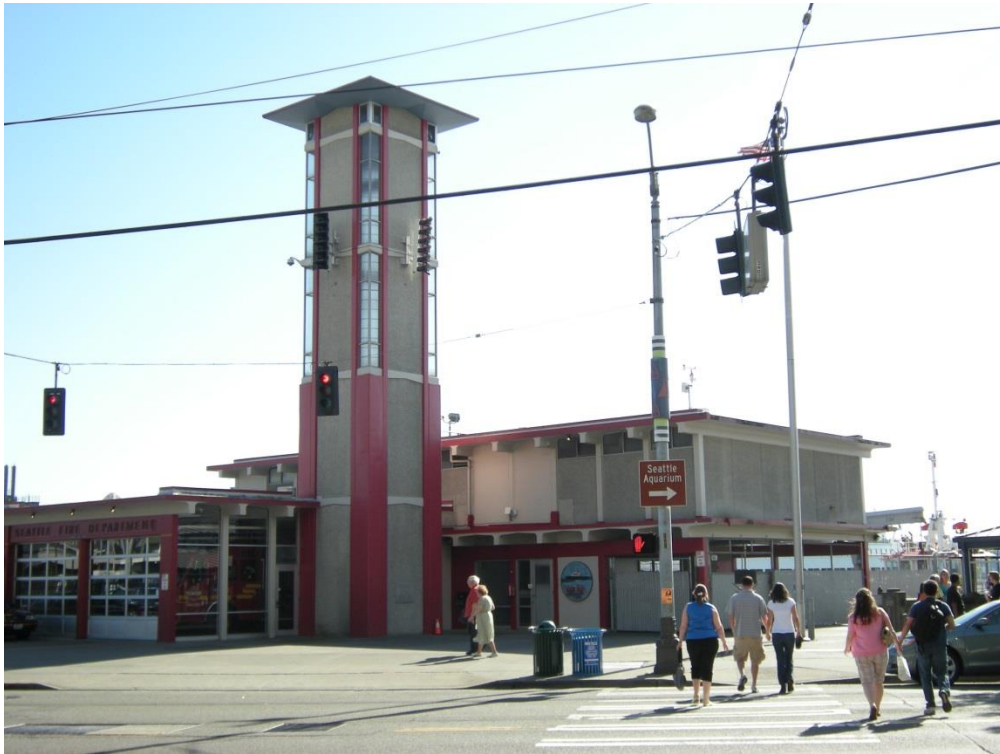
Fire Station No. 5, 925 Alaskan Way, current
