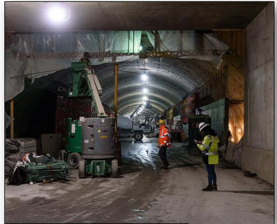
Work on the southbound (upper) roadway of the SR 99 tunnel
