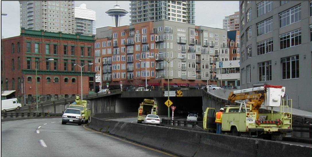
Battery Street Tunnel during a semiannual inspection
