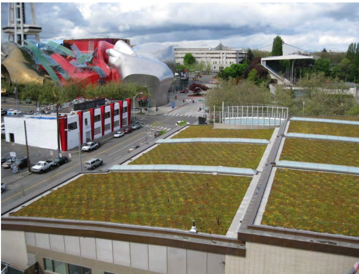
Large Green Roof, Seattle, WA
