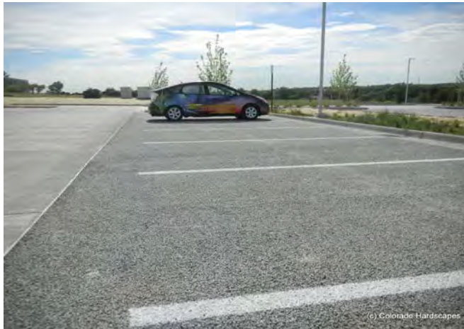
Example Porous Concrete
