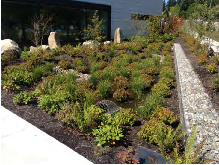
Example of Small Bioretention Facility, Edmonds, WA
