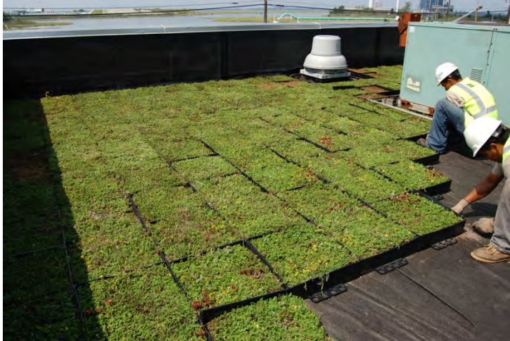
Green Roof Retrofit, Seattle, WA
