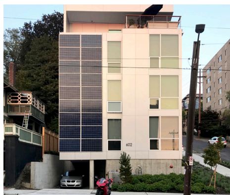
Solar panels add interest to facade and help meet the buildings energy needs.
