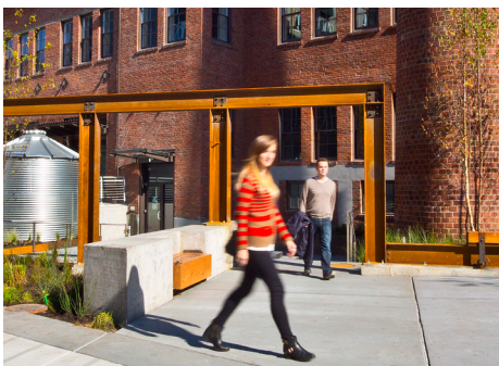
Reclaimed lumber from the adjacent historic building have been repurposed into landscape elements.
