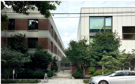
New construction mimic the scale and massing of the existing streetscape while using contemporary materials and window patterns.
