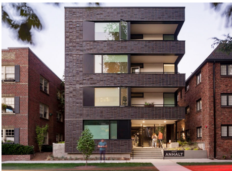
Traditional brick is used for a contemporary modern design.
