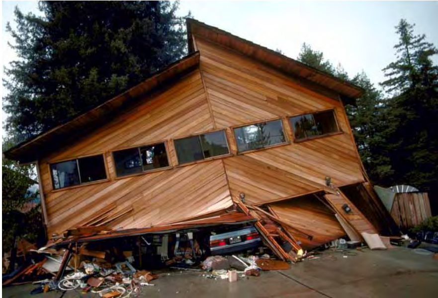
Figure 5-8. Home Damage Due to Inadequate Cripple Walls
