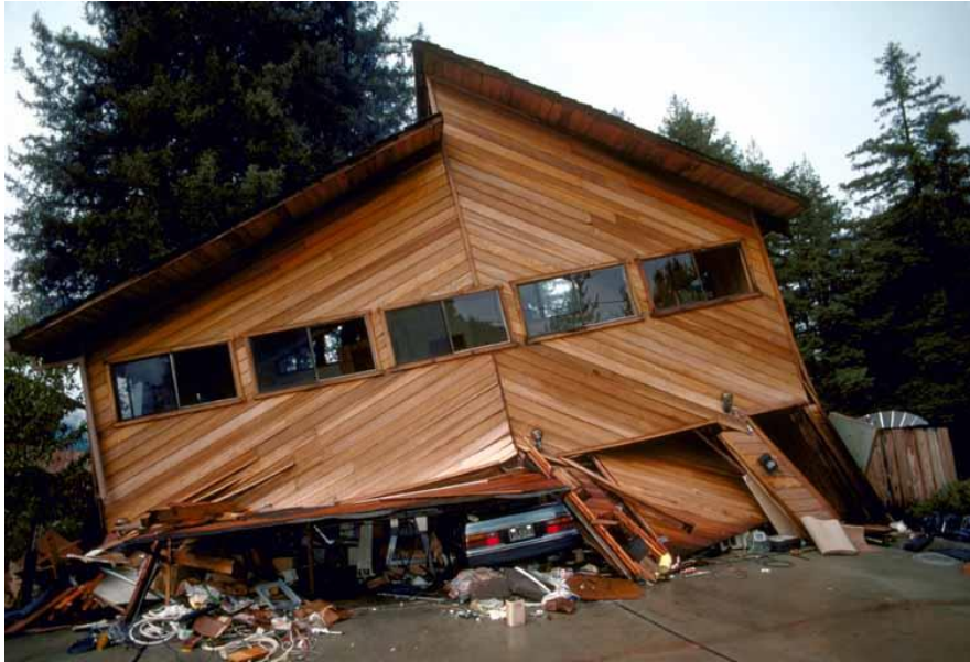
Figure 5-8. Home Damage Due to Inadequate Cripple Walls
