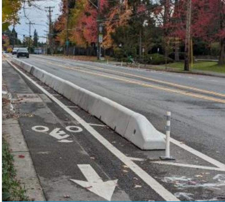
Regular bike lane maintenance and improved bike lane barriers at locations including 5th and Main to Jackson, Banner Way, and Gilman Ave W
