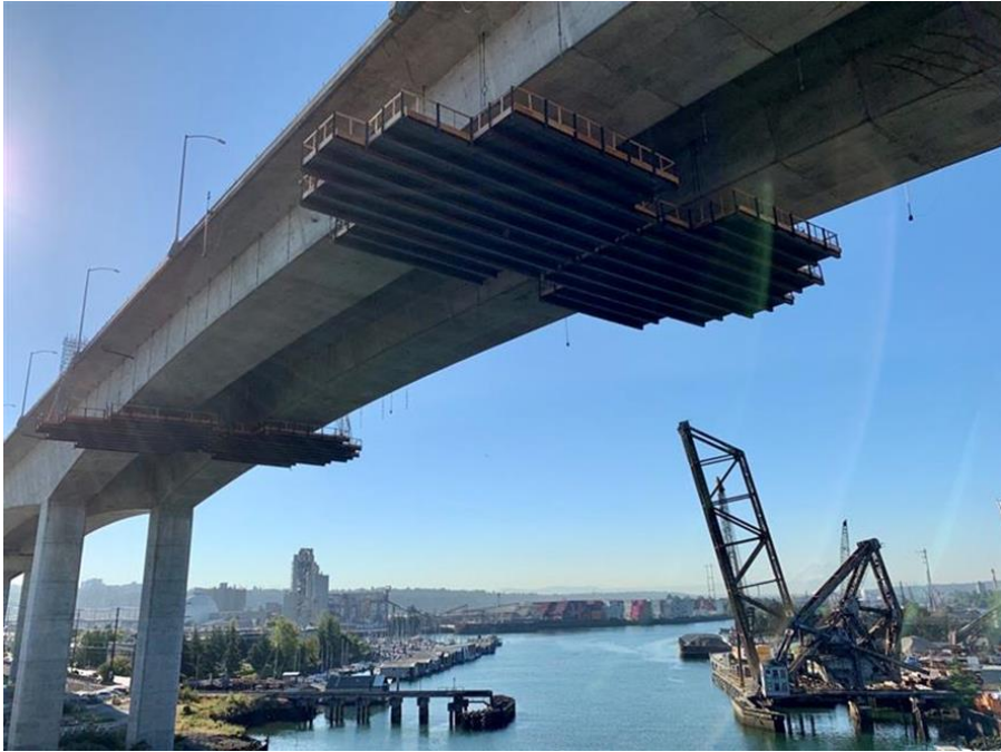
Work platforms installed in July
