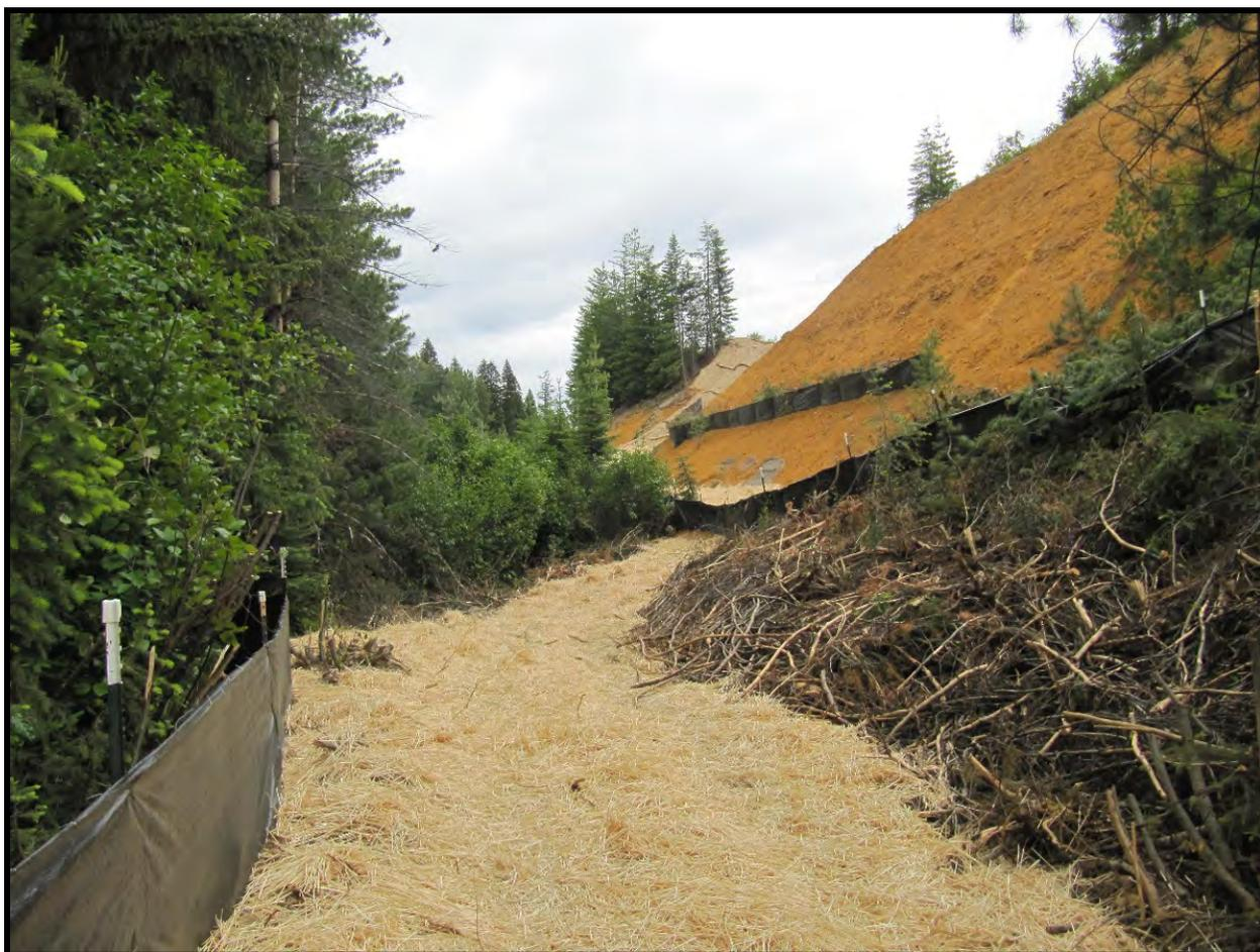
Figure 13. Filter Fence Installed on a Slope.
