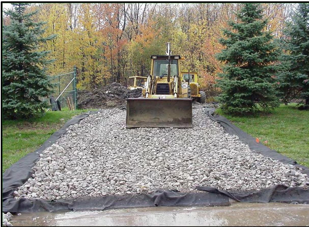
Figure 6. Stabilized Construction [Entrance Access](#).
