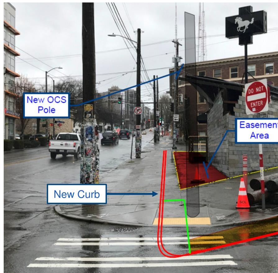
Deck at Pony has been modified to clear the easement area for Madison BRT construction
