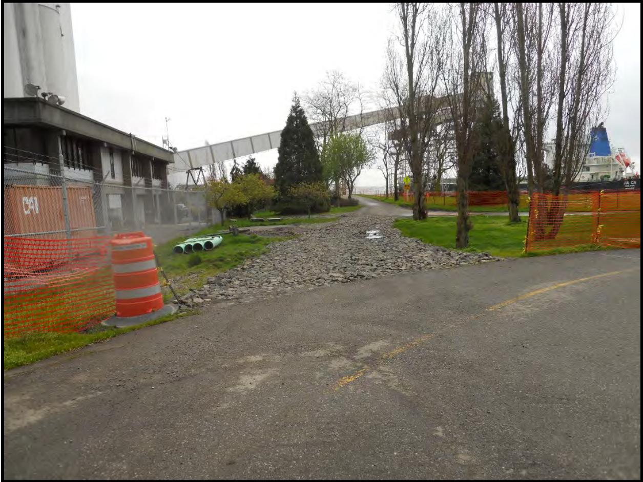
Figure 7. Stabilized Construction [Entrance Access](#).
