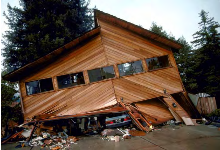
Figure 5-8. Home Damage Due to Inadequate Cripple Walls
