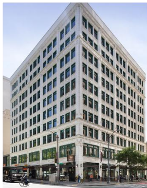
Joshua Green Building, 1425 4th Ave Seattle
